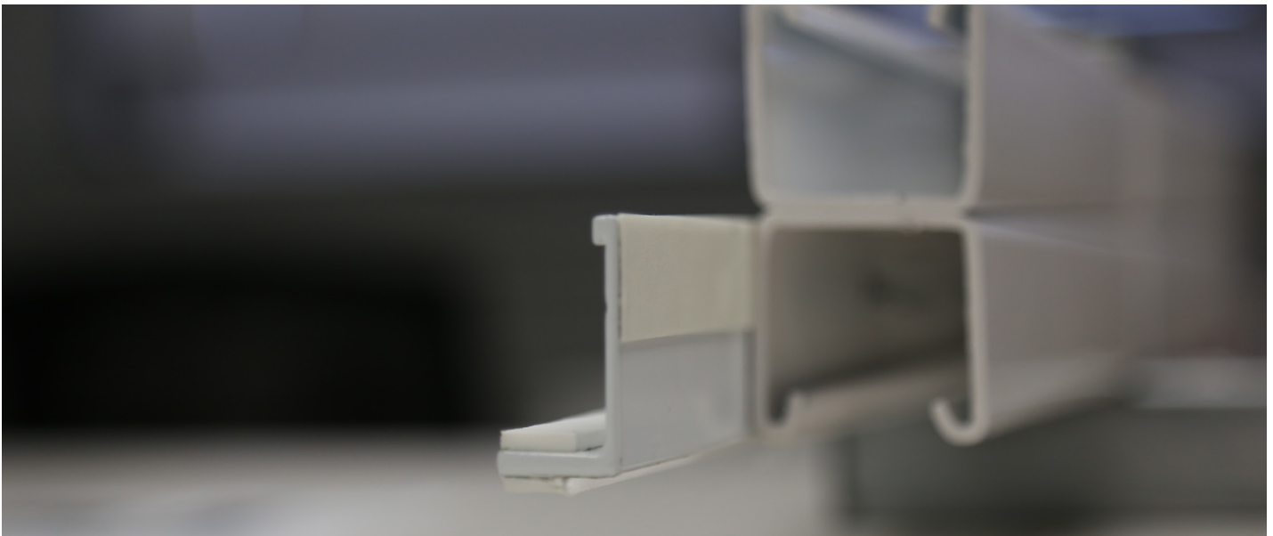
Figure 12. Installed 1/8 in. x 1/2 in. (Part Number 042373-002) on Room Side of Price Half Tee
