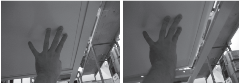
Figure 25. Removal of Ceiling Access Panel
